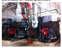
Jordan's Furniture has two Direct Fire Absorber Chiller for Cooling and Heating. The cooling tonnage capacity 1287 USRT.
