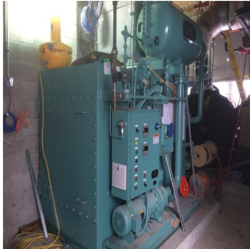
Heat Recovery Steam Generator (2,245 lbs/hour )
