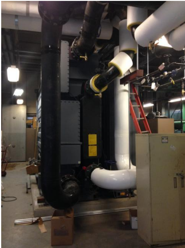
Absorption Chiller (350 Ton)
