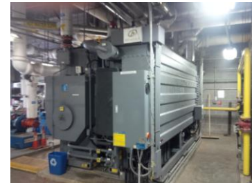
Con Ed Plant has 2 BZ Direct Fired Absorption Chillers
