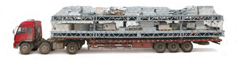
During assembly, the prefabricated columns are erected and the floor plates are simply fitted into position, making the construction process "as easy as playing with Lego". The role of the on-site workers is mainly just to connect the steel columns, bolts and wall panels, and to link up the pre-installed wiring and piping between the plates.
